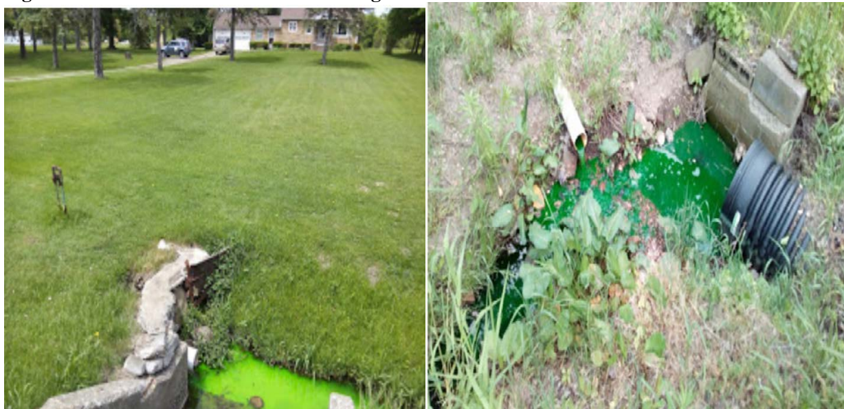
Figure 7: Pictures of confirmed illicit discharges
